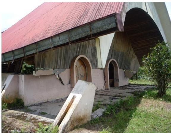
Figure 3. Damage on Cinchona Church after earthquake 2009.
